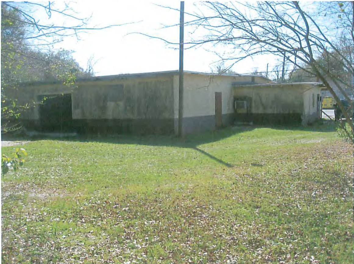
Rear View of Subject Office/Warehouse Building
